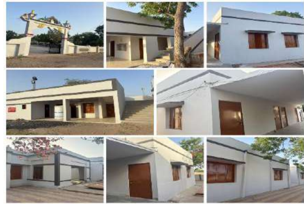
School Renovation - Bhuj
